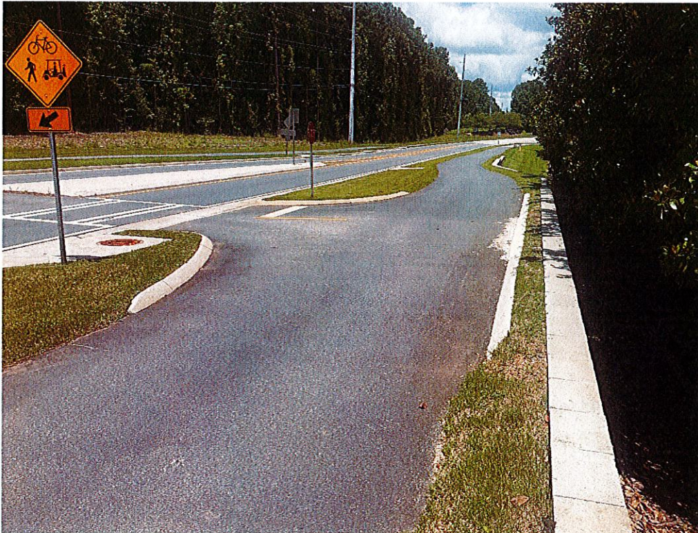
Photo 1: Section of sod between header curb and retaining wall to removed
